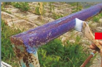
Apply SABI Change after the surface preparation (SP3).
