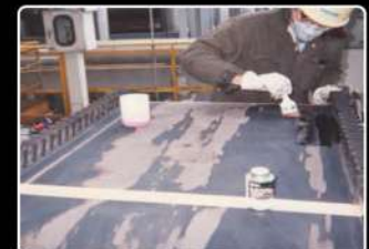
Repair of conveyor belts for coal transport
