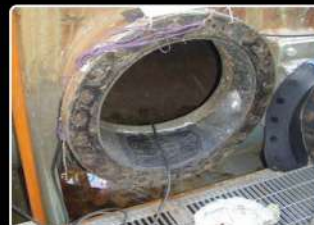
Repair rubber lining of circulating water pipe manhole
