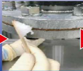
② Apply on leakage area
