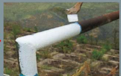
After drying, overpaint with general paint.
