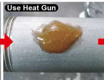
Apply after warming up the repair area and turn to gold after 20 min heating.
